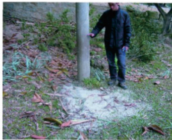
(e) 喷砂冒水与电线杆下沉
