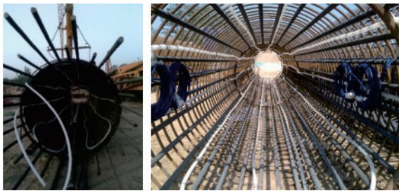
(a) U行管布置 (b) 传感器及感应线布置
