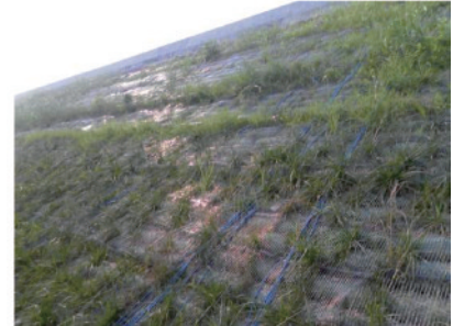
图4 竣工后的加筋路堤 Fig.4 the reinforced embankment
